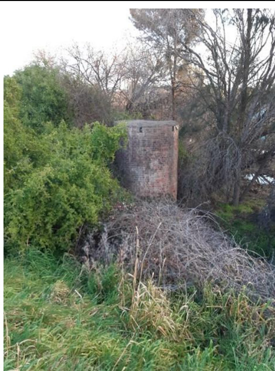
Figure 8: Shaft B (tunnel air shaft) east side of Macquarie River weir
